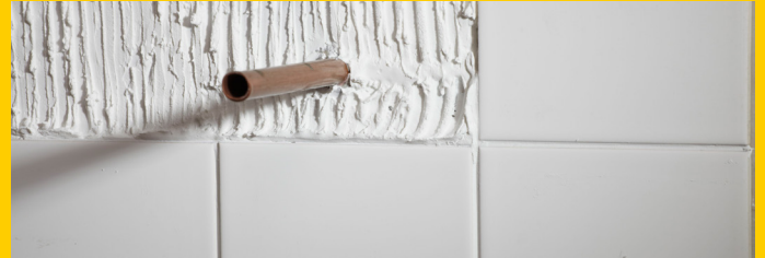
22. REPLACING DAMAGED TILES
