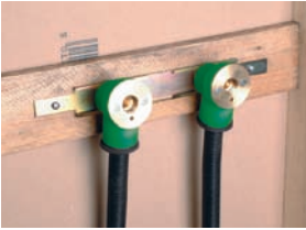
Fig. 48 HX101/15, 15mm conduit terminal and HX103 terminal back plate
