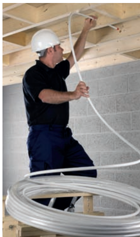
Fig. 22 Packaging retains pipe until last metre
