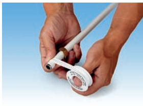
Apply PTFE tape if required
