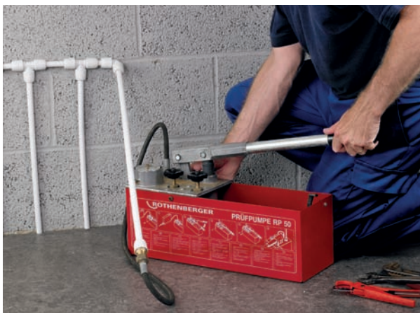
Fig. 59 Pressure testing
