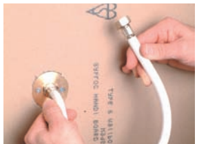
Fig. 50 Installation of HX102 terminal fitting plate and HX101/15, 15mm conduit terminal
