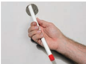
Fig. 23 Always protect pipe ends
