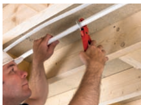
Measure and cut in-situ
