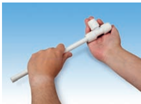
Fig. 11 Hep 2 O jointing sequence
