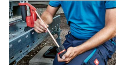
2. Deburr and remove all external sharp edges.
