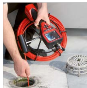
Inspection of rain downpipes
