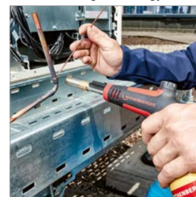
Brazing in refrigeration / air-conditioning technology
