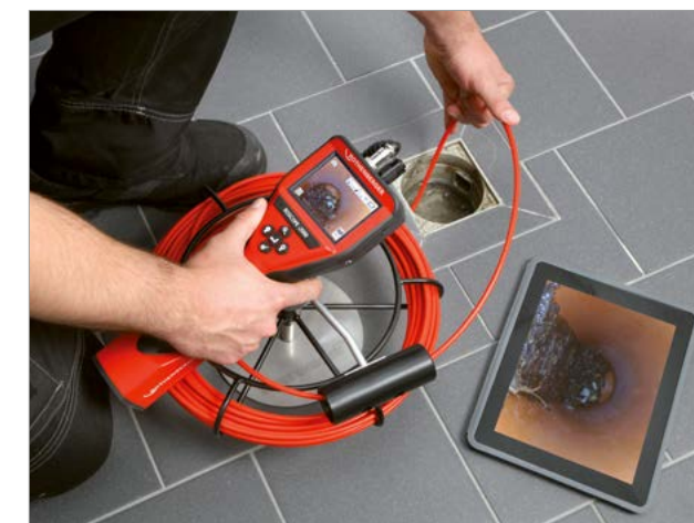
Inspection of basin drains
