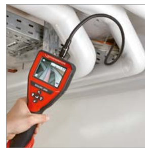
Inspection of hollow spaces
