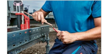
3. Use a pencil deburrer on internal edges.
