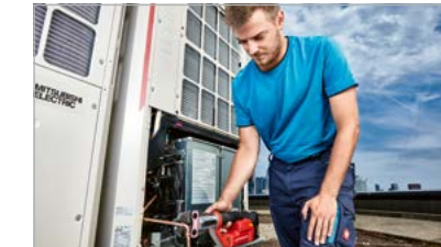
8. Align jaws squarely on the fitting and complete the joint.
