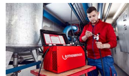
The use of heat conductive paste guarantees optimal freezing
