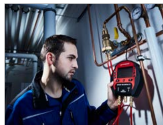
Pressure and leakage testing for gas pipelines according to TRGI 2018
