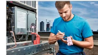
7. Mark insertion depth using depth gauge and insert tube fully into the fitting.
