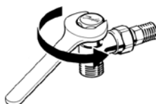
Removal of protective cap
