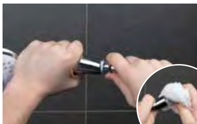
Unscrew your existing shower head from the shower hose and discard old washer. Clean threads on shower hose.
