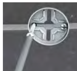
Screw 'X' plate to the wall
