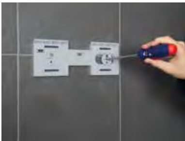
FIX Fix the bracket to the wall and adjust the level.
