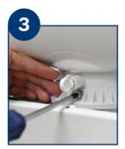
Attach the Greenstar Xtra to the adaptor using the included unit fixing screw.
