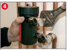
Loosely secure the MagnaClean Professional canister to the valves. Grip the MagnaClean canister and tighten the compression fittings being careful not to over tighten.
