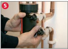
Loosen off the valve flange nuts and insert the rubber washers provided. Thoroughly tighten the flange nuts. Do not over tighten. Refill the heating system.
