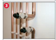
Prepare the pipe and fittings accordingly. Lubricate the olives and assemble the valves on the pipe. Hand tighten.
