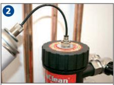
Wait for five seconds before removing the adaptor. The Pro-Fill air vent will accept all market-leading chemicals in either liquid or concentrate form.
