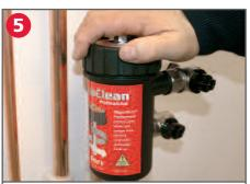
Replace the lid assembly onto the canister and tighten until sealed. Do not over tighten.
