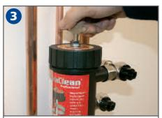
Replace the Pro-Fill air vent. Allow the system to circulate for 30 seconds. Open the Pro-Fill screw two turns and back flush until clear.
