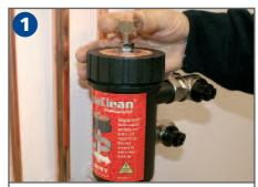
With a standard radiator key remove the Pro-Fill air vent. The built-in, one-way valve will prevent water from escaping. Attach chemical adapter and feed in chemical.
