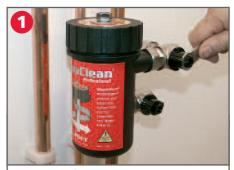
Important – Before commencing any servicing work, turn off electrical supply to the boiler. Ensure the water is not too hot to undertake work on the system. Turn off both isolation valves to the marked OFF position. Loosen the air vent to release internal pressure. When venting, protect the surface below the canister with a dust sheet or container to capture any drops of water.
