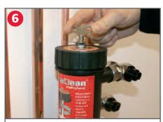
Open the isolation valves to the marked ON position and vent/bleed through the Pro-Fill air vent. Protect the surface below the canister with a dust sheet or container to capture any drops of water. Run the central heating system while checking for leaks. Repeat steps 1 - 6 if required. Ensure the filter is thoroughly clean before leaving the premises.
