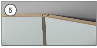
Starting at approximately 45°, angle the tongue of the next panel into the groove of the fixed panel. Ensure the tongue is fully inserted into the groove before snapping it back to the wall, otherwise it may damage the joint.
