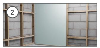
Bond the first panel to the wall or frame, with the grooved edge first. If screw fixing panels to the wall/frame, pilot bore the recess in the groove where screws are to be located. (failure to pilot bore may result in the panels splitting). Pack between back of panel and wall as necessary to avoid distortion to the Hydro-lock joint when screw fixing.
