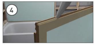
Apply masking tape to the two meeting edges of the decorative face to protect the laminate face. Apply a narrow bead (2-3mm) of silicone sealant to the front shoulder of the tongue.
