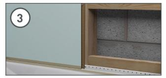
Fix through the back flange of the grooved edge with countersunk screws - the screw head should fit into the recess on the back of the tongue. Ensure that screws are turned until they are just under the flush to prevent any obstruction to the tongue of the next panel to be fitted.
