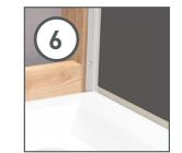
Apply adhesive to the reverse of the panel, angle into the first profile and push firmly against the wall.
