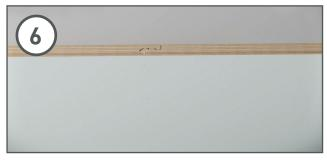
Remove the masking tape and ensure any excess silicone sealant is wiped from the laminate face immediately.
