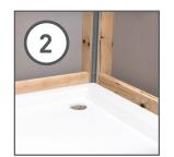
The first profile, normally start with an Internal Corner or End Cap, should be fixed to the wall or end grounds with countersunk screws, or adhesive and a bead of silicone sealant applied to the channel
