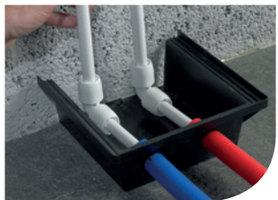
Figure 40: Cut conduit box for wall termination
