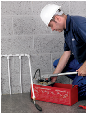
Figure 59: Pressure testing
