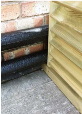
rear slot detail for pipework and cables
