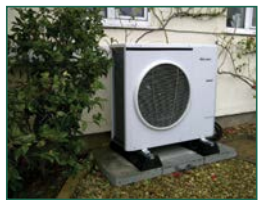
5. Secure the ASHP units onto the kit - the installation is complete.
