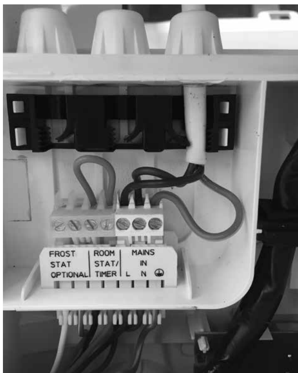
INSTALLER CONNECTIONS (LHS)
