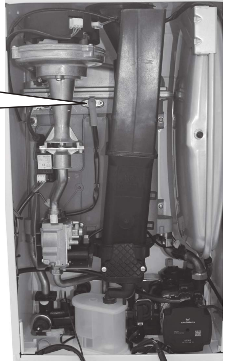
Flame Detection Electrode
