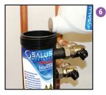
Pour a bottle of water treatment corrosion and scale inhibitor, we suggest SALUS Inhibitor. The canister will hold 500ml.
