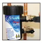
Open the isolation valves and start the heating system.
