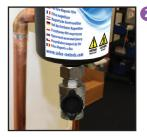
Close drain valve using drain cap, ensure the cap is alligned correctly so the valve is fully closed.
