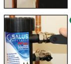
Open inlet to flush out debris.
