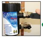
Important – Before carrying out any servicing work, turn off electrical supply to the boiler and let the water cool down to a safe working temperature. Using the Mag Defender spanner provided turn both isolation valves to the OFF position.
