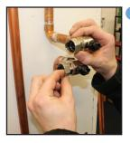
Now Loosen off the valve flange nuts and insert the rubber washers provided. (There are 2 supplied with this product).
