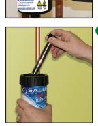
Remove magnet and put in a safe place.
