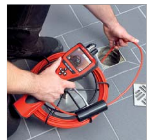
Inspection of floor drains
