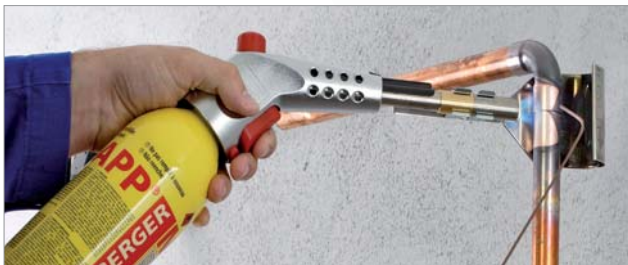
Brazing in gas installation
