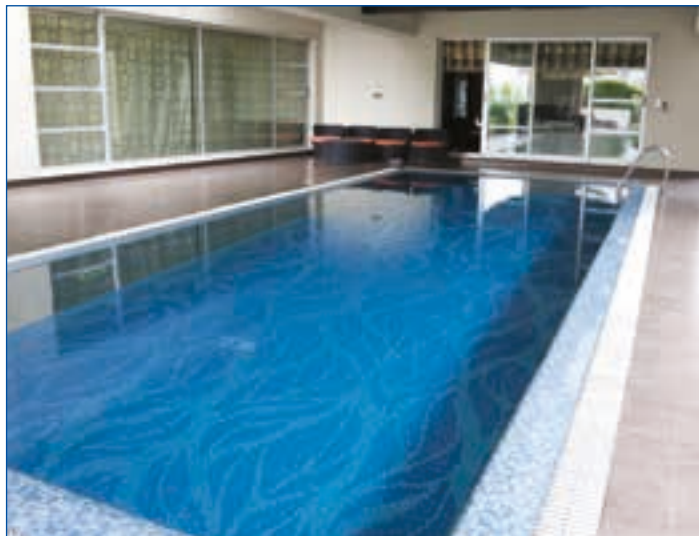
The Greenstore LECP ground source heat pump can be used to heat swimming pools
