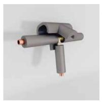
Insulate as far as the T shape. Make the T shape (with inside diameter = outside diameter of the insulation), apply it and stick firmly.
