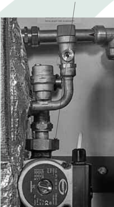
Figure 4-4: Removing flow & return pipe
