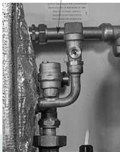
Figure 4-10: Re-fitting flow & return pipe
