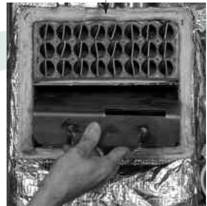
Figure 4-7: Removing baffles from boiler shell
