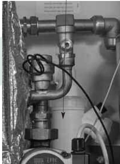
Figure 4-12: Re-fitting condensate trap
