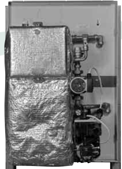
Figure 5-2: System boiler Flow and Return connections
