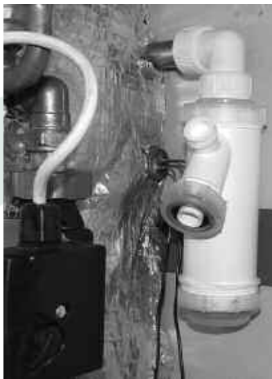
Figure 6-3: Condensate trap
