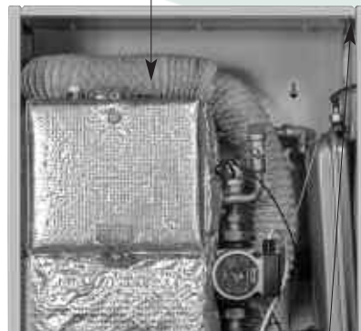
Figure 4-2: Dismantling the boiler
