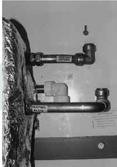
Figure 5-1: Non-system boiler flow and return connections
