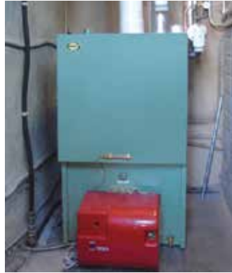
Model shown: Grant Vortex Pro 46-58kW Boiler House model installed in a cellar
