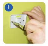
Attach the wall mounting bracket to a suitable wall using the fittings supplied and the built in level.
