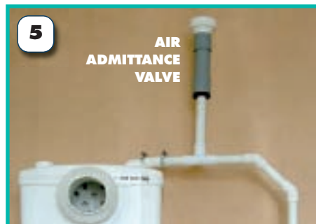
7 Where the pipework falls to a floor lower for example, fit an air admittance valve at the highest point capable of withstanding 10psi pressure, or increase pipe size coming down to 'break' syphon.
