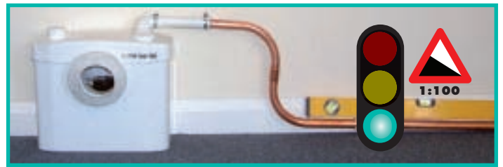
2 Discharge pipework should be copper or rigid solvent weld plastic, not 'pushfit'
