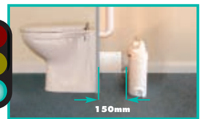
10 If boxed in, the boxing should be easily removed. Any extension between the WC pan spigot and wall should not exceed 150mm.
