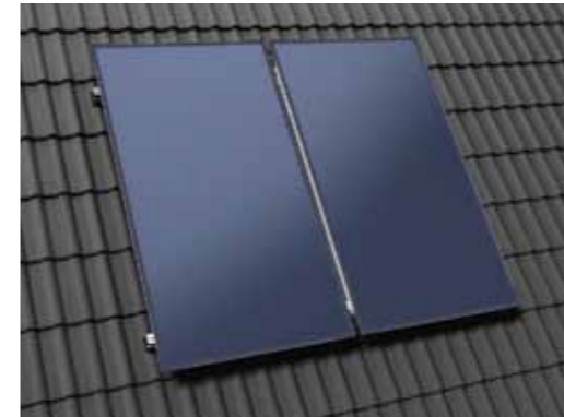
Solar-Lifestyle on-roof installation
