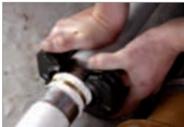
Gripping the pressing collar with intermediate jaws
