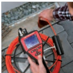
Inspection of rain drainage pipes
