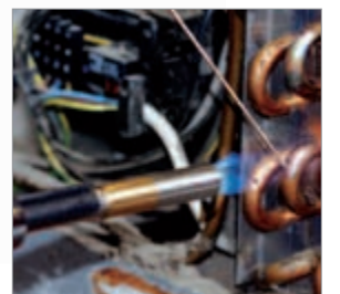
Hard soldering in refrigeration and climate control
