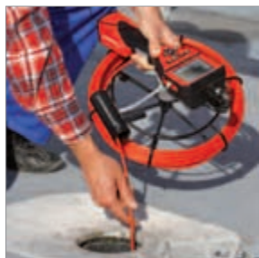
Inspection of rain downpipes
