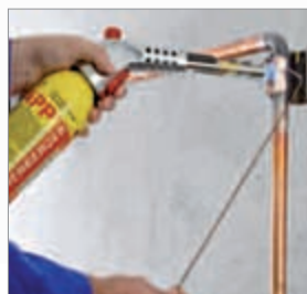
Brazing in gas installation
