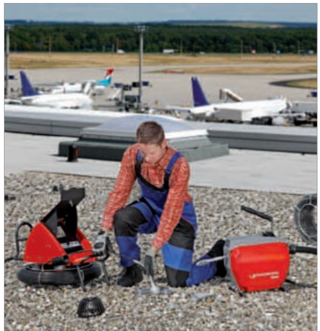
Inspection of a rainfall drains
