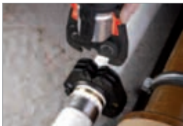
Gripping the pressing collar with intermediate jaws
