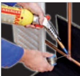
Soft soldering in heating installation
