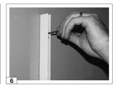
Drill holes into wall using 7mm masonry drill bit. Fit wall plugs provided or fixings suitable for the construction of your wall. Fit channel using three No. 8 x 30mm long Pan Head Pozi screws provided. *Figs. 7.1, 7.2 & 7.3*
