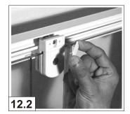
Using 2.5mm allen key, position and fix door stops in top and bottom frame to prevent the sliding door banging into the wall frame.
