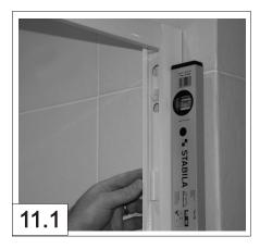
Check the door frame is level, vertical and square on all sides of the unit. Fig.11.1 Frame **must not** be twisted or buckled when fitting. Use the adjustment screws as described in stage 5, if necessary.
