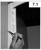
B Detach connector posts from wall frames and re-position these to marks made on walls. Using spirit level to ensure posts are vertical, mark through 3 pre-drilled holes in each post. *Figs. 8.1 & 8.2*
