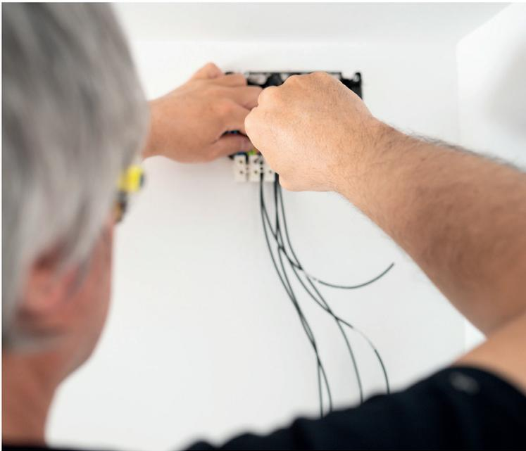
The E7+ comes with an adaptor plate for retrofits. This allows fresh installations to be more ergonomic and streamlined, whilst still making the E7+ a plug in replacement for all the existing legacy water heaters from Horstman - Electronic 7 and Economy 7 Quartz.
