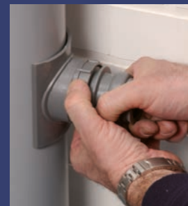
4. Twist in the Easy Boss connector
