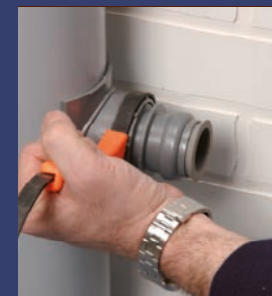
5. Use a strap wrench and hand tighten
