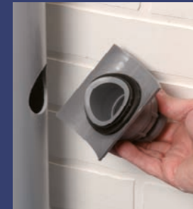
2. Ensure seal is in position
