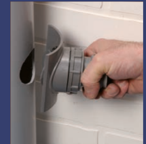
3. Insert Easy Boss into hole
