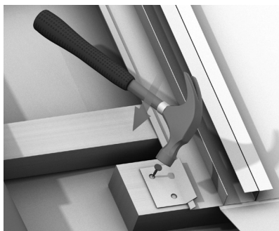
Figure 6-18: Securing Side Gutter Clips
