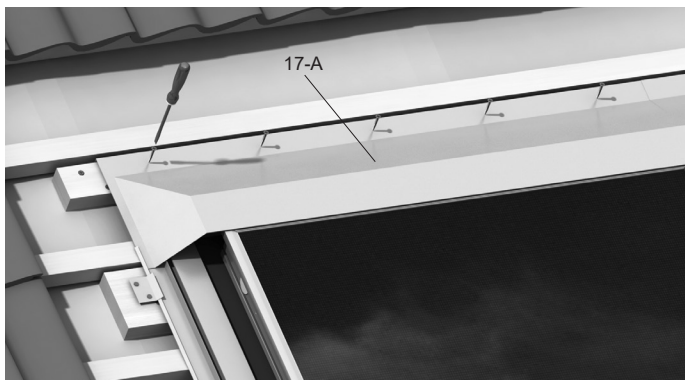
Figure 6-28: Fixing left hand Top Cover Flashing (17-A)
