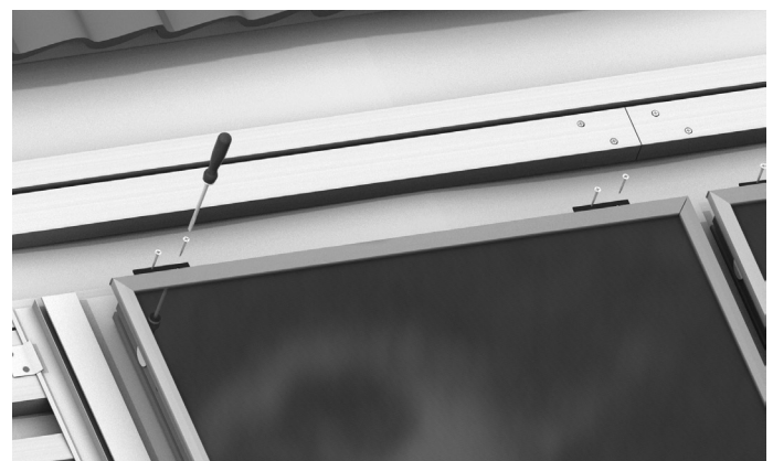
Figure 6-26: Fixing of the Top Brackets
