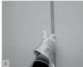
3 Remove plasterboard. NOTE: The vapour barrier must not be damaged!
