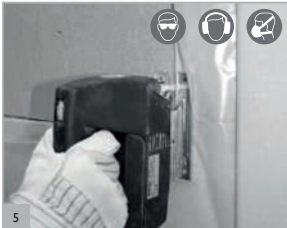
5 Make the opening. NOTE: Load Bearing elements must not be weakened! IMPORTANT: follow the safe working notes on p.35.
