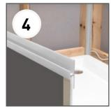
Apply silicone sealant to the channel of the second profile and attach it to the long edge of first panel.
